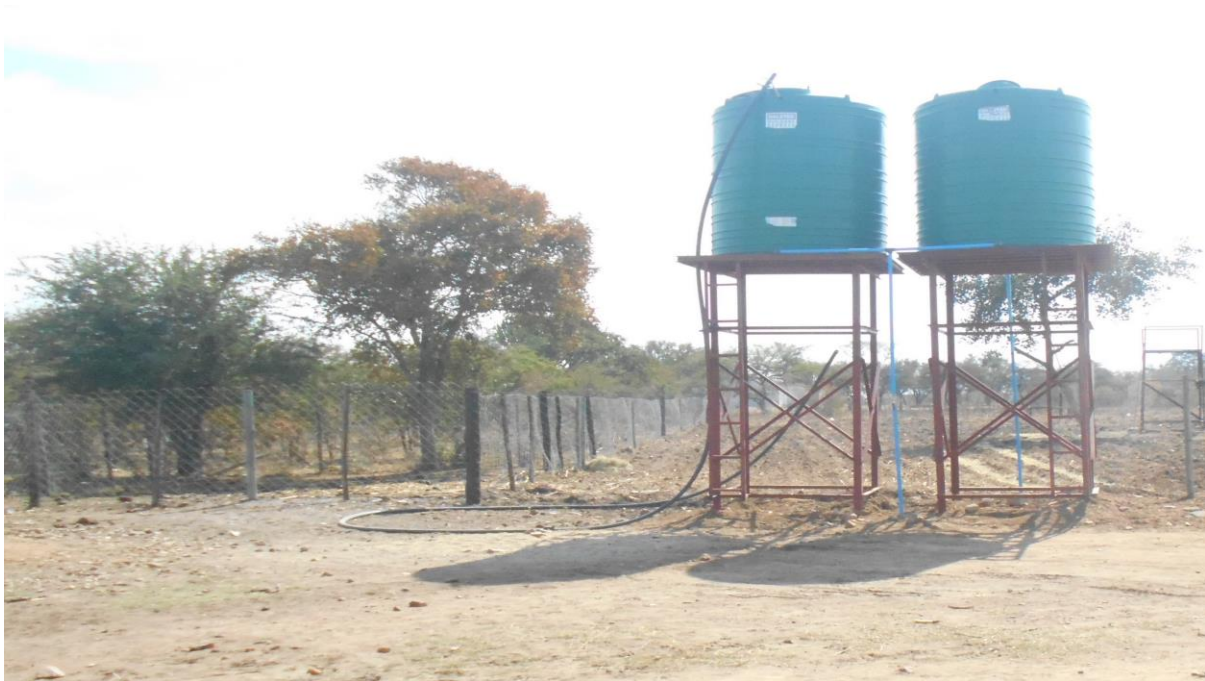
THE 2x5000 LITRES WATER TANKS FOR TRANSFIGURATION CHIDZIKWE YOUTH SKILLS TRAINING CENTRE
