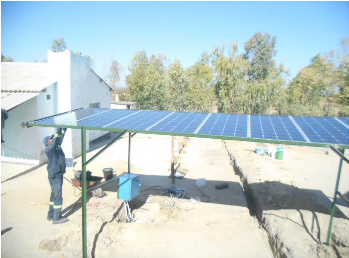
ELECTRICIAN FITTING SOLAR PANELS FOR PUMPING WATER INTO WATER TANKS AT ST. BONIFACE MISSION.
