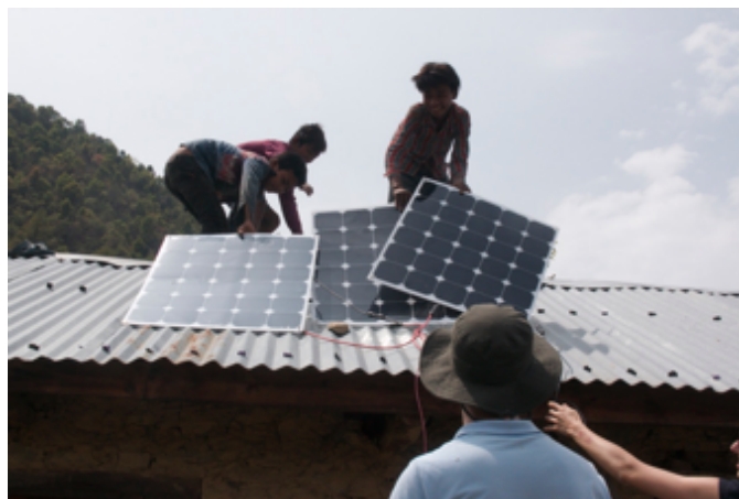
Bijay (our engineer), Suman and helpers Installing solar panels on the school-roof
