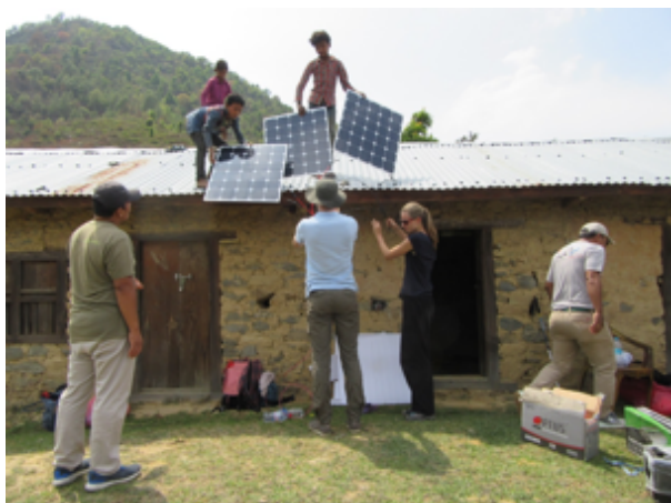
Bijay (our engineer), Suman and helpers Installing solar panels on the school-roof
